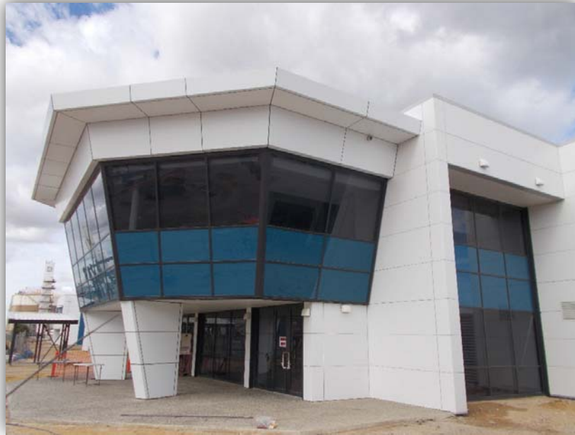
Figure 2 - Non-Process Infrastructure Control Room at Kwinana
