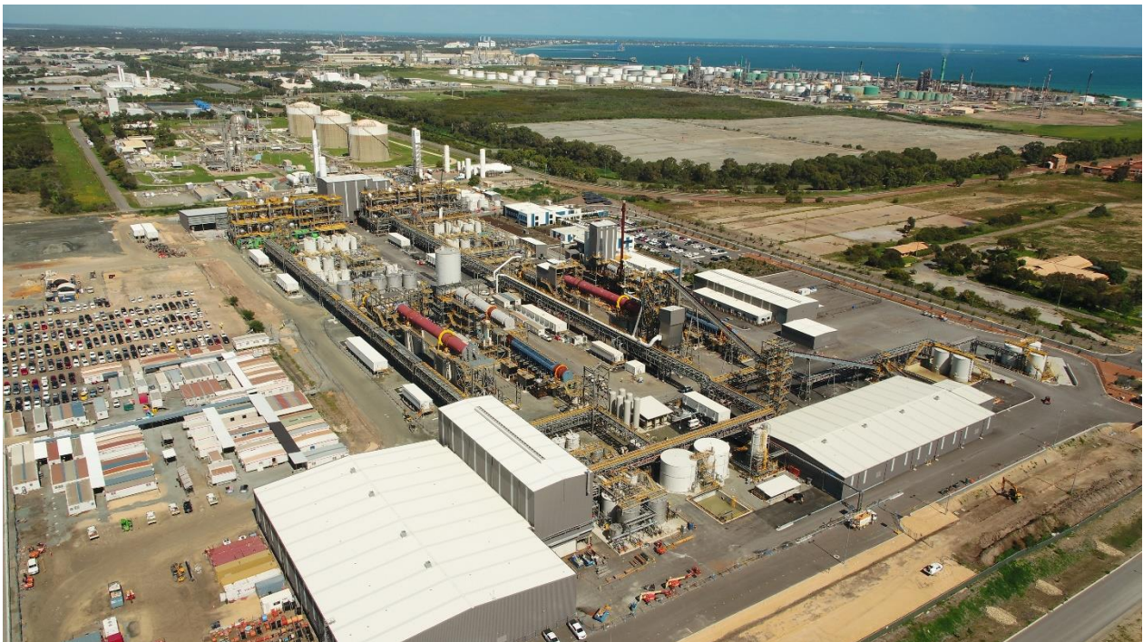
Tianqi Lithium Australia's Lithium Hydroxide Production Plant at Kwinana, Western Australia.
